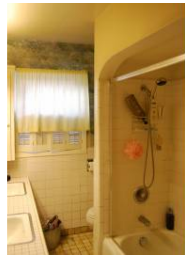
BEFORE: A NE Portland bathroom remodel by Michael Howells
